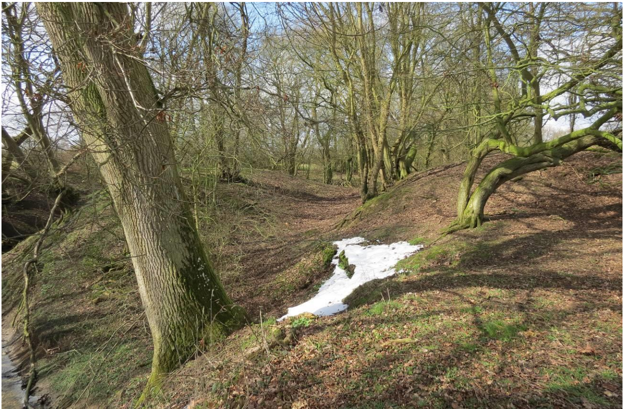
Figure 14: The spillway site viewed from south of the dam.
