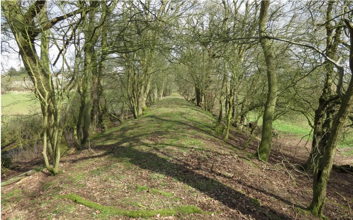
Figure 4: The top of the dam, looking north east.
