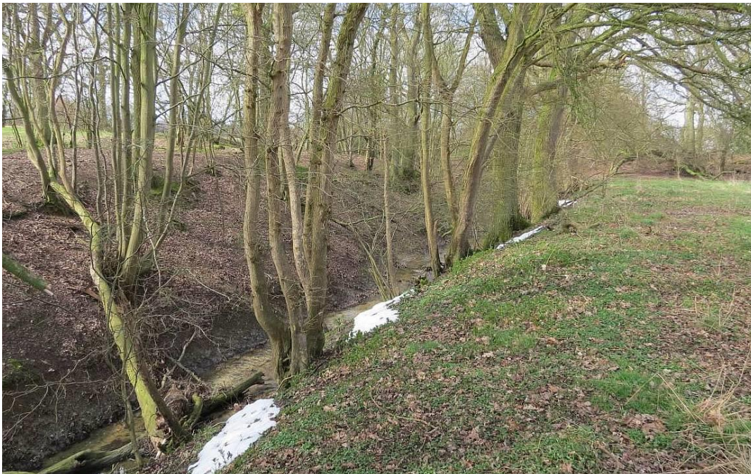
Figure 16: The channel immediately downstream of the dam.
